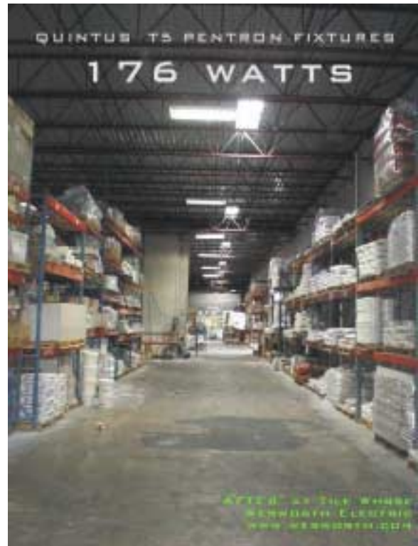
AFTER: Notice that these new Quintus fixtures 1) produce a constant light level on the floor 2) illuminate the sides of the shelves 3) render a clear crisp light overall 4) SAVES 60% WATTS! and 5) PAID FOR ITSELF WITHIN 2 YEARS!
